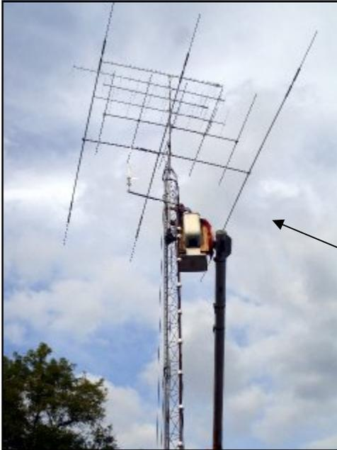
This is the installation of my Cushman A3S 3 EL Beam and cable support system.
